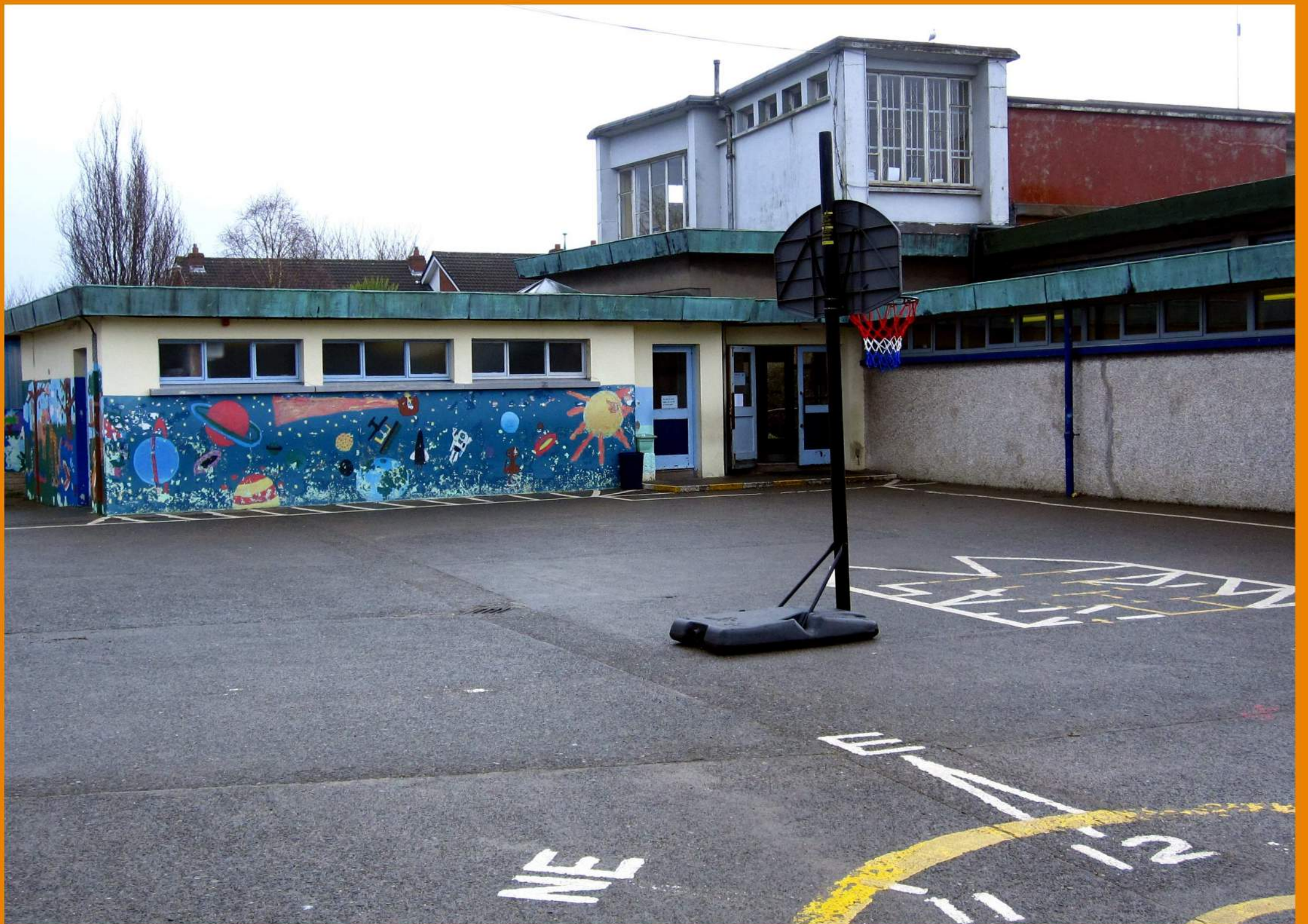
This is the old yard just before the demolition began.
