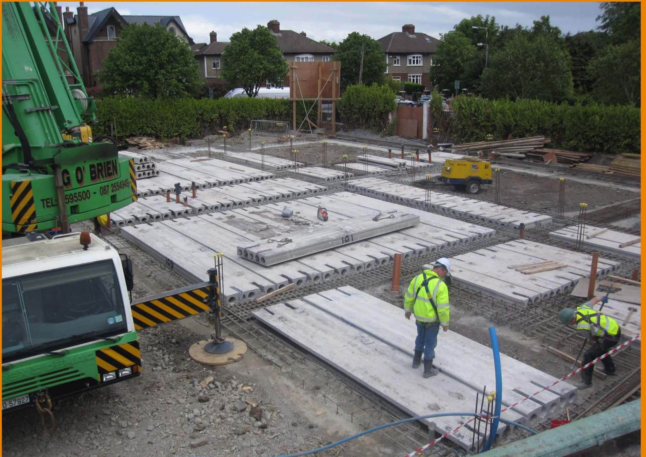
Foundations are laid and the building begins .....
