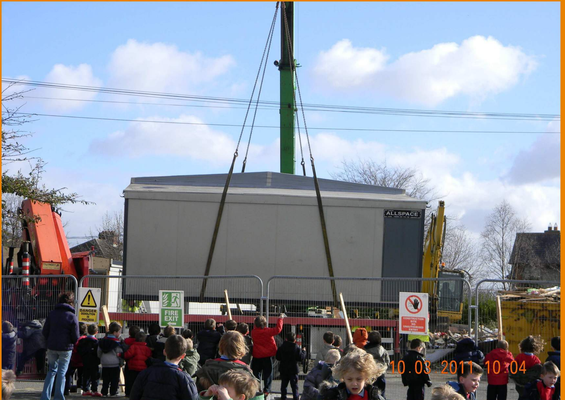
Making way for demolition .....
